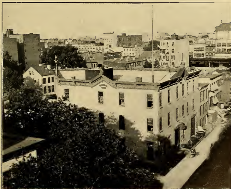
WESTERN END OF CHURCH LANE. [Arrow points to wall running on center line.]
